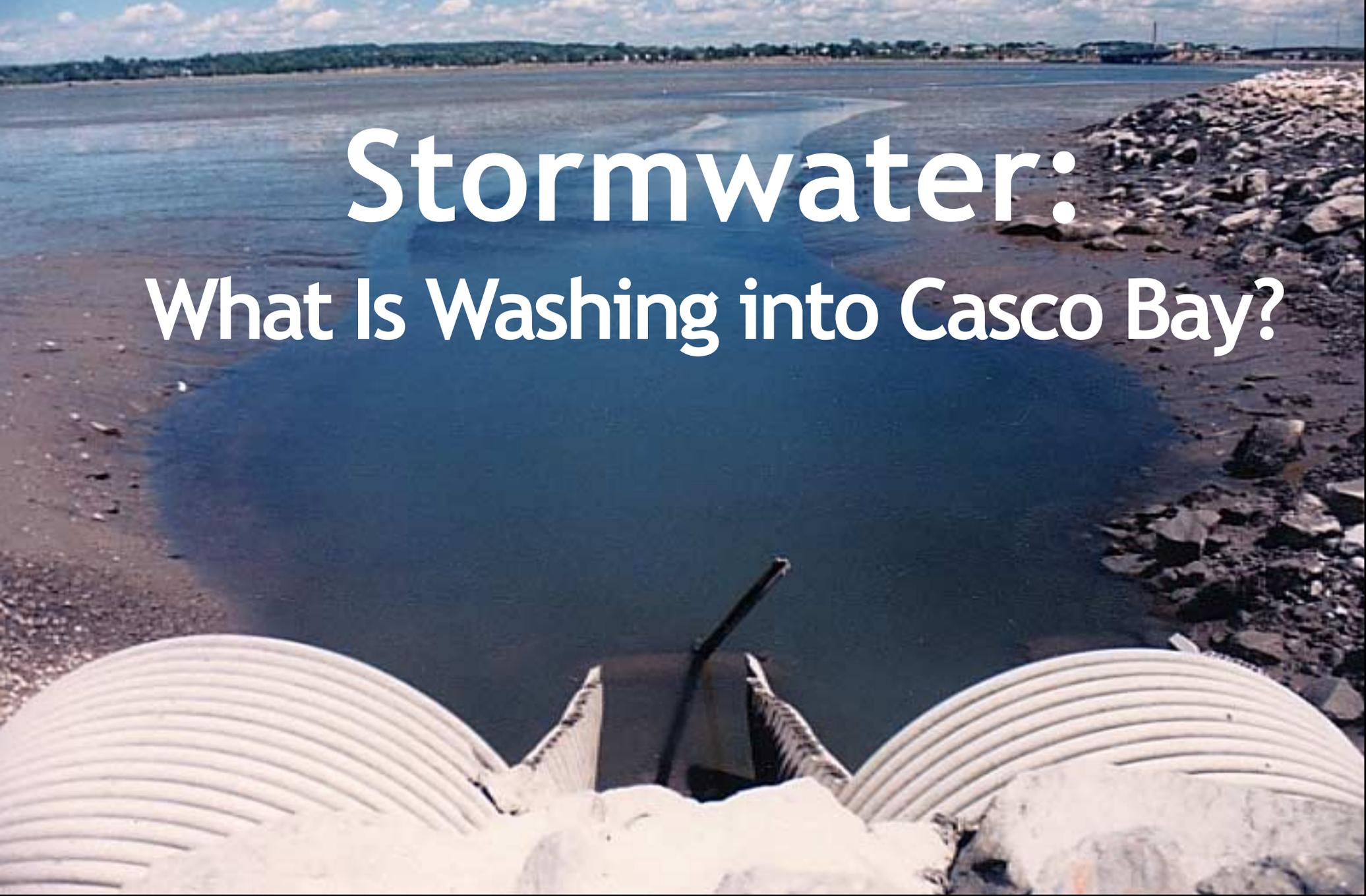
*During heavy rains, untreated municipal wastewater can flow directly into Casco Bay through outlets like these combined sewer overflow pipes along Portland's Back Cove.*
