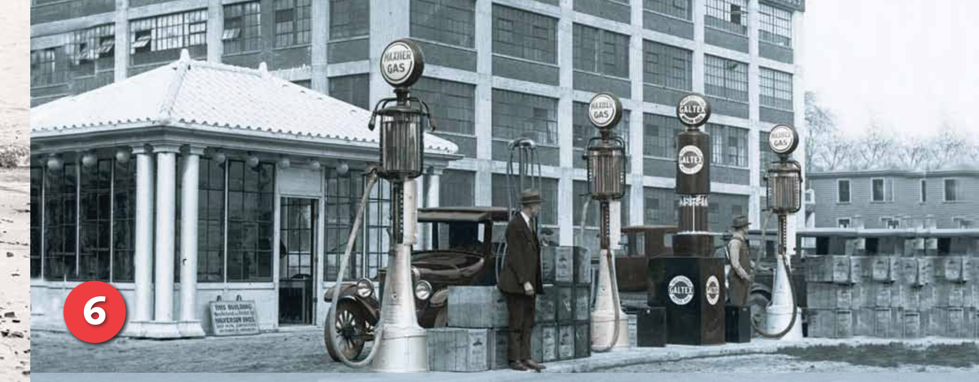
6 As GAS STATIONS grew common in the 1950s, GASOLINE full of toxics began leaking from corroded tanks into the groundwater, then into the Bay — an ongoing, sometimes hidden, problem.
