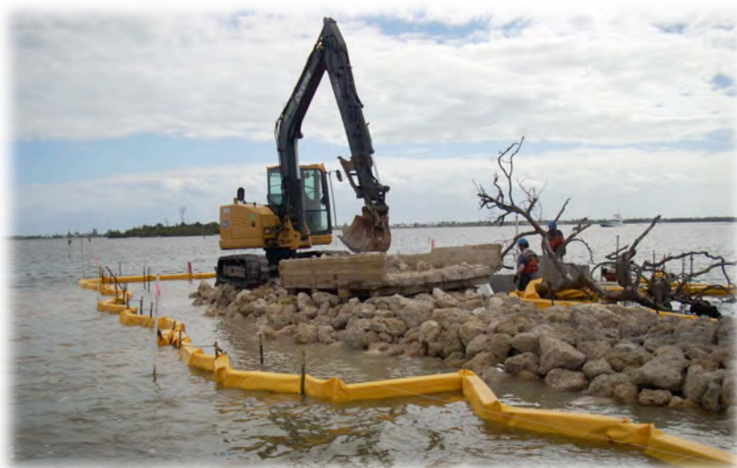
Figure 19: Wave break installation at Bird Island /Photo: USFWS
