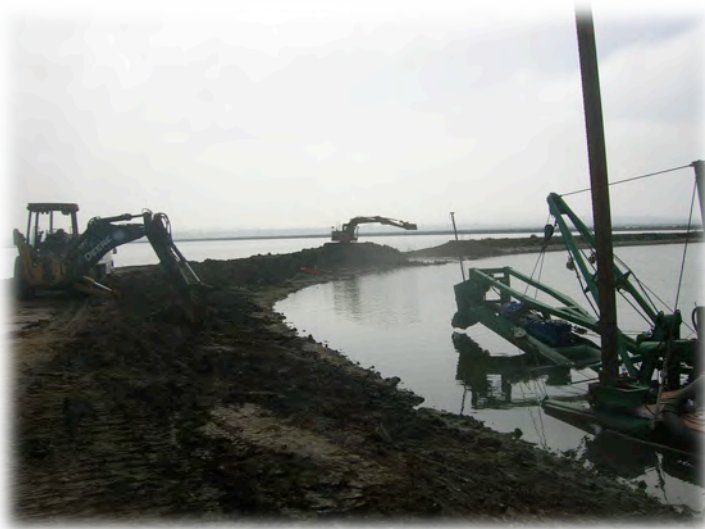
Figure 25: San Diego Bay Levee breach to reconnect waterway / Photo: USFWS
