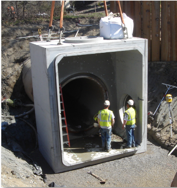
Baxter Boulevard CSD storage conduit during installation.
