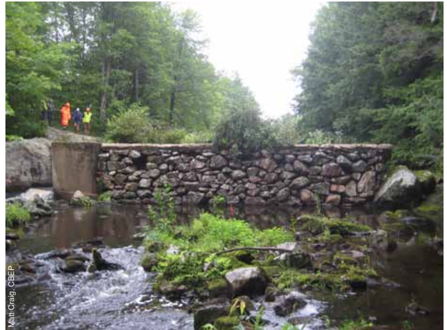
In 2013, Trout Unlimited, working closely with private landowners and Caribou Springs, LLC, removed Randall Mill Dam on Chandler Brook (a tributary to the Royal River), with support from CBEP, USFWS Gulf of Maine Coastal Program, Maine Rivers, Royal River Conservation Trust and others. A dam had been on the site since 1796.
