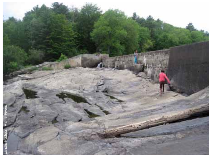
Bridge Street Dam in Yarmouth, one of two dams that span the lower main stem of the Royal River, sits just one-third of a mile upstream from head of tide, disconnecting the Royal River watershed from Casco Bay.
