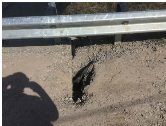
Erosion at 9079 documented on 4/25/16 (photo: Wright Pierce)
