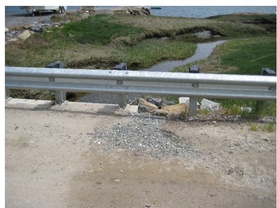
Repair by landowners, documented on 5/25/16 (photo: CBEP)
