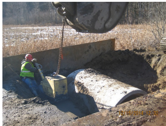
Figure 1. Installation of open bottom concrete box culvert IN December 2014 at the lower site (9079, left) and embedded concrete round pipe at the upper site (9078, right).
