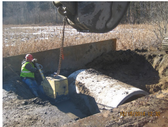
Figure 1. Installation of open bottom concrete box culvert IN December 2014 at the lower site (9079, left) and embedded concrete round pipe at the upper site (9078, right).
