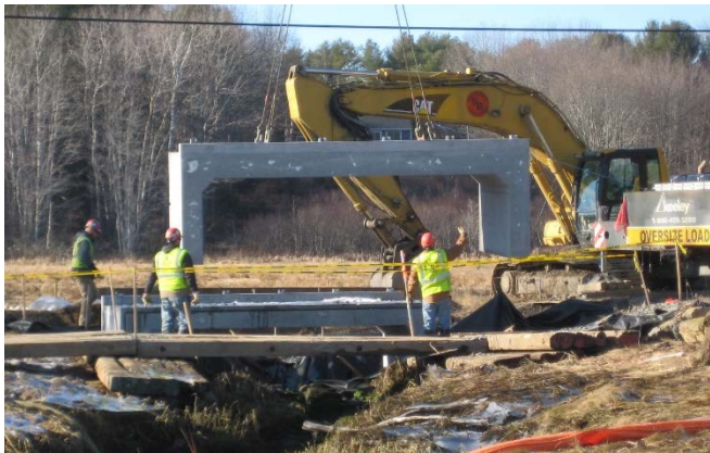
Figure 1. Installation of open bottom concrete box culvert IN December 2014 at the lower site (9079, left) and embedded concrete round pipe at the upper site (9078, right).
