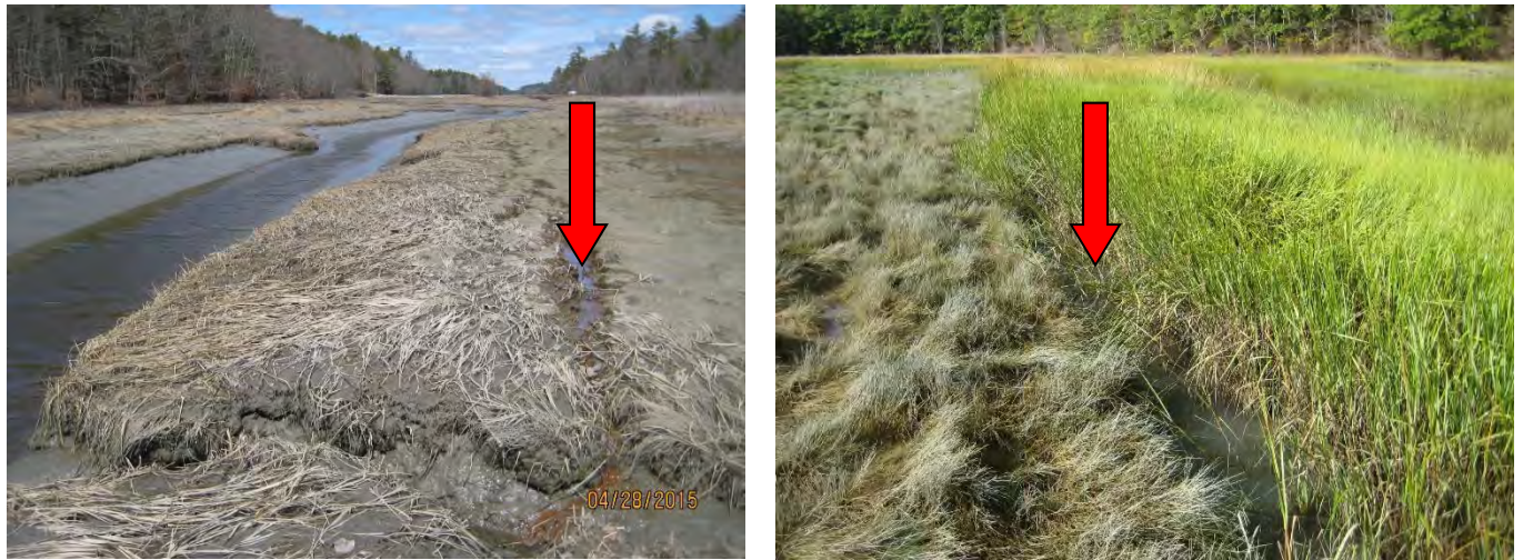
Figure 35. Photos: channel edge near St 4 showing expanding rill, indicative of ongoing channel erosion.
