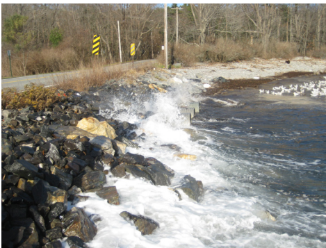
Waves ripple into Pond Cove Brook through the culverts under Shore Road in Cape Elizabeth. The road experiences splash-over with increasing frequency during astronomical high tides and winter storms.
