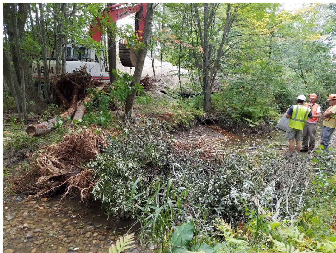
Long Creek contractor and design team reviewing the project plans as they construct a log jam in the Main Stem of Long Creek in South Portland. Photo: Long Creek Watershed Management District
