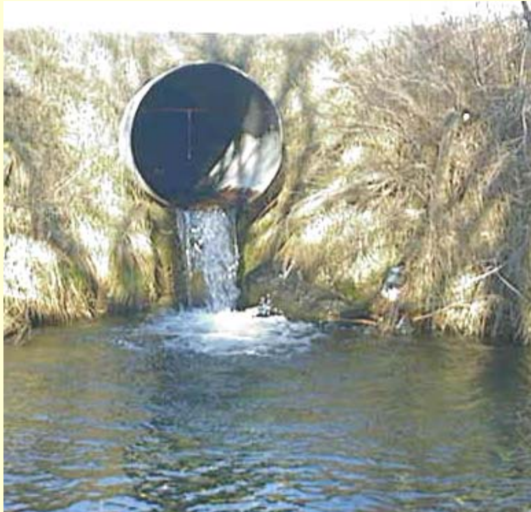
Scour downstream of undersized Culvert-ANR Photo
