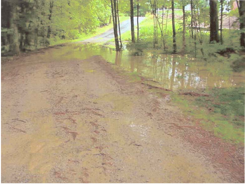
Figure 3: Flooding across Whippoorwill Lane August 2003
