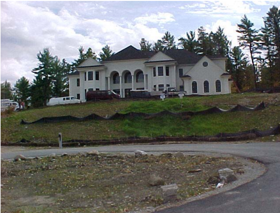
Figure 5: House with 8000 square feet impervious area on Burgundy Terrace
