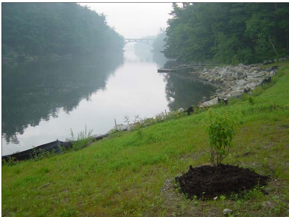
June 2006. Presumpscot River southern shore facing downstream at site of Smelt Hill dam removal. Note willow waddles planted during fall 2005 flourishing in front of silt fence along the length of the site.
