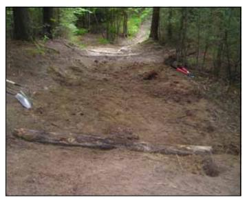
Trail runoff was causing severe erosion on this steep trail section in Blackstrap Preserve. The crew measured and cut timbers that were on site and installed the waterbars to divert runoff to small plunge pools and vegetated areas. The crew also leveled out the soil and reinforced the timbers with rocks to help slow the runoff further and allow infiltration.
