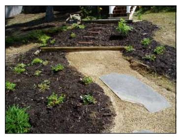
This path from the landowner's backyard to the lake was eroding due to foot traffic and stormwater runoff. The YCC installed an infiltration landing, planted a variety of shrubs and groundcovers and secured landscape timbers across the path to divert runoff into a vegetated area for infiltration. The area was also covered with erosion control mulch to protect the soil.
