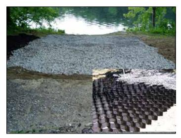
The park was planning to use this site which was experiencing severe soil erosion to rent canoes and kayaks this summer which would increase foot traffic and soil disturbance. The YCC installed 328 sq. ft. of Geoweb, providing a load distribution system that would stabilize the surface and prevent further loss of soil. Shaw Bros. Construction and Gorham Parks and Rec. Parks and Rec. provided all the necessary materials.
