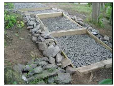
One of three sets of infiltration steps that were retrofitted at Riverbank Park by increasing the depth of the steps, filling with larger (1 1/2") crushed stone and reinforcing the edges with sidebars and riprap. Westbrook Public Works provided assistance and all the necessary materials for the work completed at Riverbank Park.
