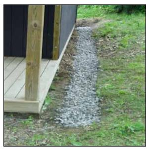
The YCC created a dripline trench to protect this structure from the damaging effects of stormwater runoff. The trench now collects runoff coming from the roof and the adjacent hillside so it can soak into the soil and not end up in the nearby Presumpscot River.
