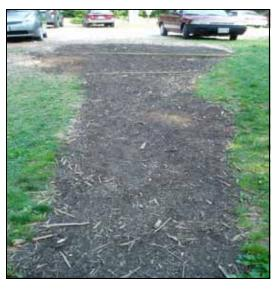
This path leading from the parking lot to the beach was washing out every year due to stormwater runoff. The crew spread 14 yards of erosion control mulch and installed waterbars at the top of each path to slow down and infiltrate the runoff. Windham Parks and Rec. supplied all the materials for completion of this project.
