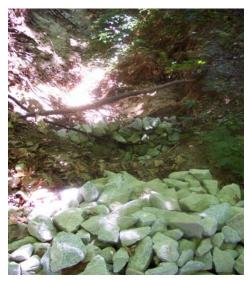
This site involved a paved turnout causing a gully to develop over a 50' slope, ending in a drop-off into a larger gully. The crew began with 20' of erosion control matting and then covered the remaining 30' with 8" rip-rap, interspersed with small check dams. At the drop-off a dam was created and a small settling basin was dug into the bottom of the larger gully.
