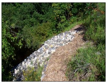
This area around two large culverts is commonly used as a fishing spot, but the culvert and surrounding soil was completely exposed (directly above this spot is a very busy section of Route 302). A 200' path leading to the spot was completely mulched and the exposed culvert and soil was armored with 6-8" rip-rap provided by Windham Public Works.
