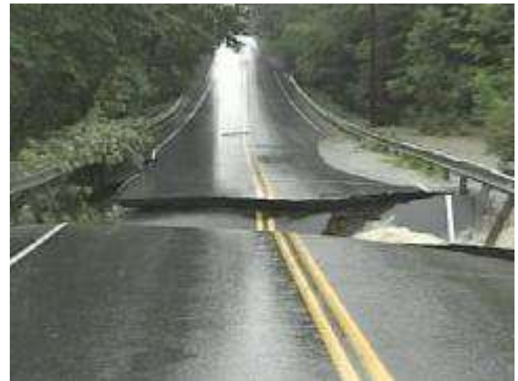
Desert Road culvert failure, Freeport August 8, 2008
