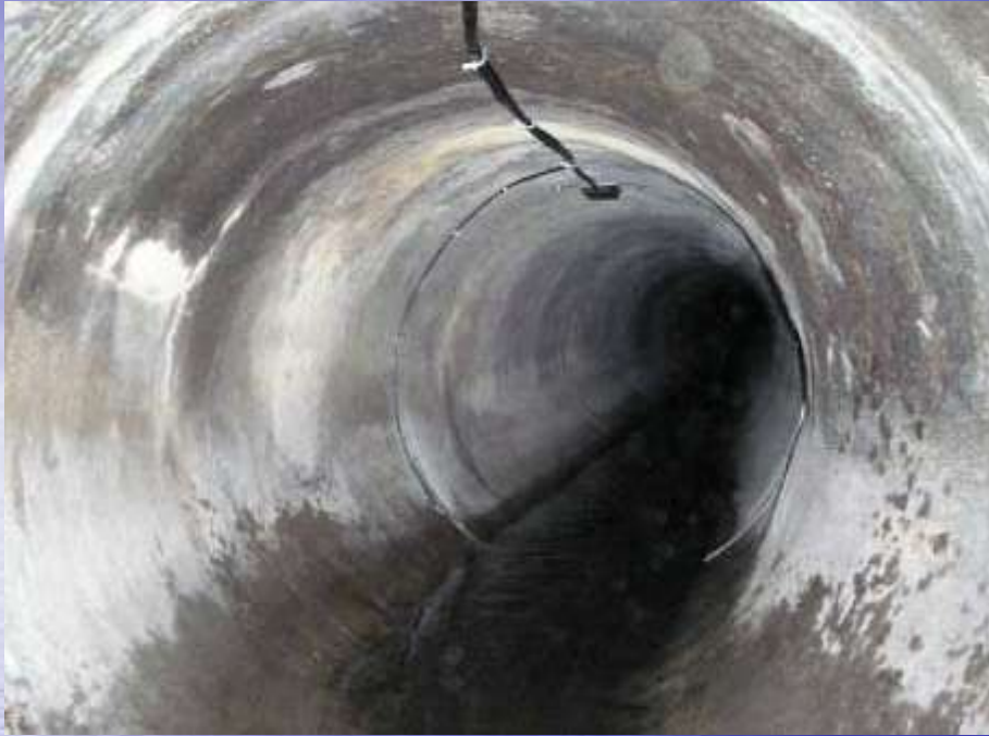
Ultrasonic Depth and Velocity on incoming flow
