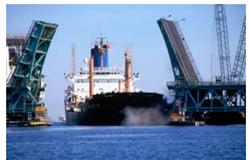
In 1996, the Julie N oil tanker spilled almost 180,000 gallons of fuel oil into the Fore River after striking the former Million Dollar Bridge while entering the harbor.
