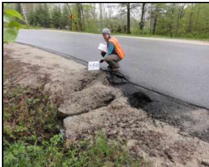
Runoff from the paved road concentrates around this culvert to contribute significant sediment to a Crooked River tributary.
