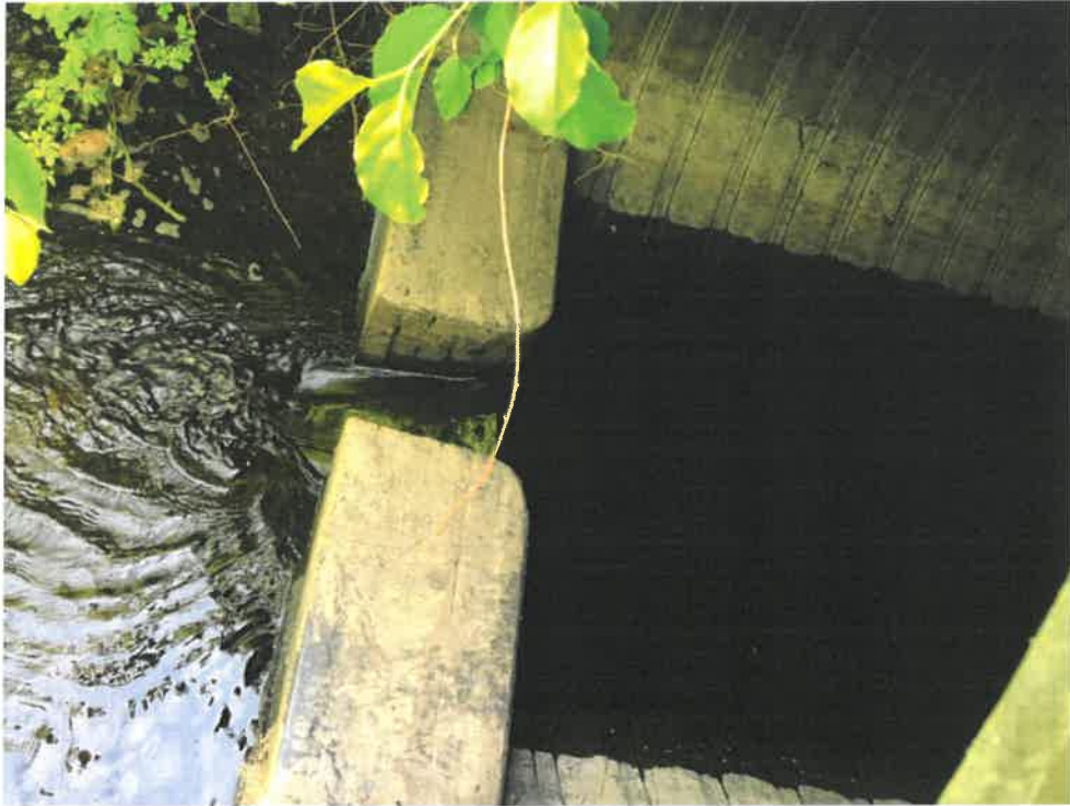
Photo 5 (06-20-18): Weir in outlet of culvert on the east side of Ocean House Road. Weir at outlet was installed to create a submerged outlet to allow Alewife fish passage.
