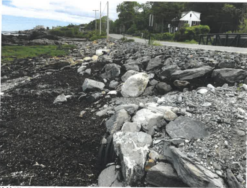
Photo 5 (06-06-18): Facing south along the rip rap armor of the oceanside outlet (west) side of Shore Road with Aluminum corrugated pipe outlet visible within the rock slope in the center of the photo.
