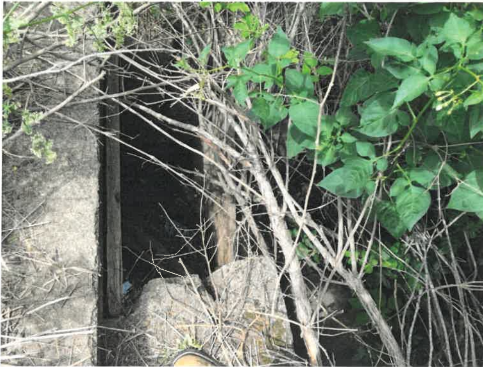
Photo 2 (06-20-18): Inlet of 36-inch High Density Polyethylene (HDPE) pipe headwall on northeast side of Sawyer Road. Concrete headwall conceals the HDPE pipe and pieces of concrete support wooden boards that creates an inlet weir to create an impoundment upstream of the pipe.
