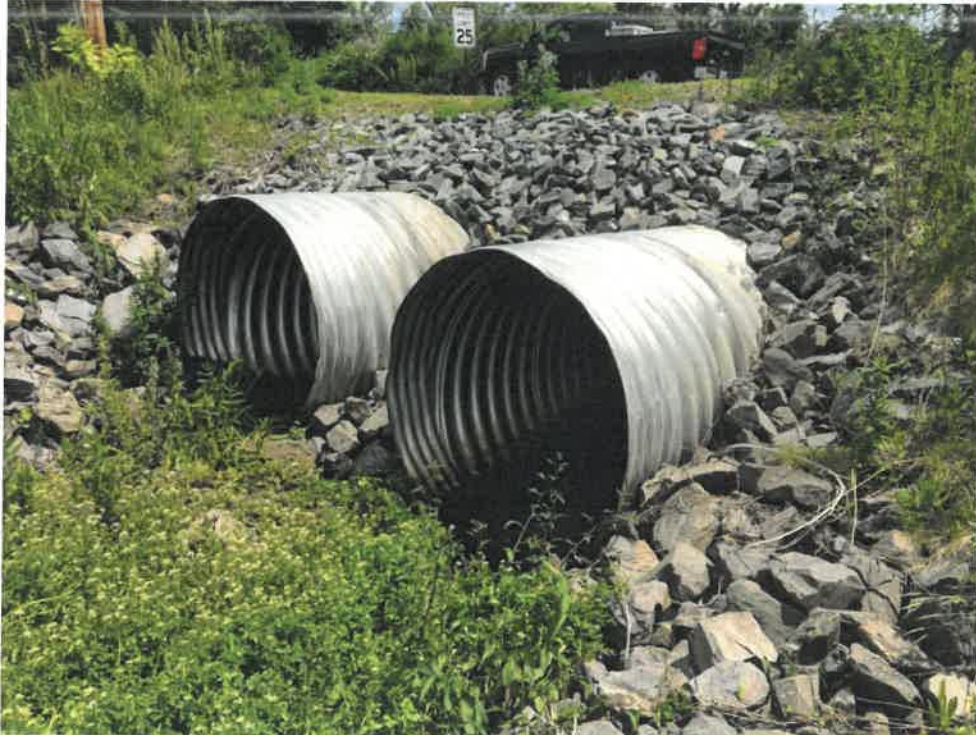
Photo 2 (06-20-18): Inlet of two, 54-inch corrugated aluminum pipes located northerly of Willow Brook. Westerly (right) pipe is set lower to carry the primary flow. Inlet has a well armored rip rap apron and headwall.
