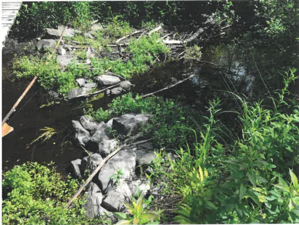
Photo 7 (06-20-18): Downstream channel of the culvert outlet flow with stone weir wall with center opening to control elevation and flow from the culverts to dissipate energy of the outfall and reduce the velocity of the outflow to the receiving channel. The weir also creates a pool area within the channel.
