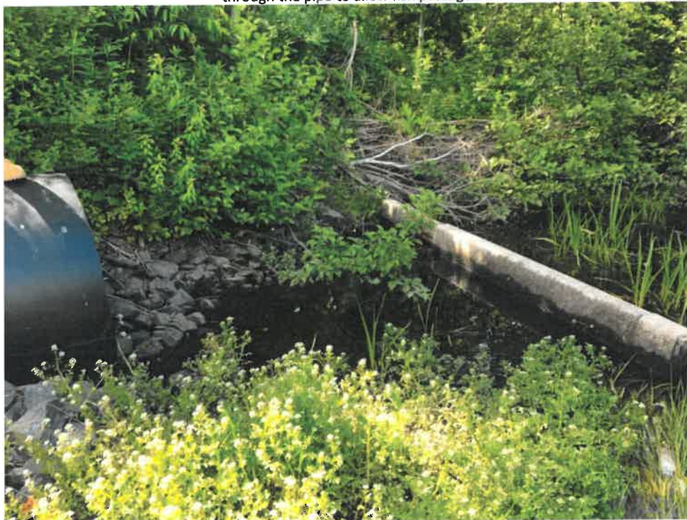
Photo 6 (06-20-18): Outlet of culverts on the east side of Old Ocean House Road. Outlet has a rip rap lined plunge pool and headwall. Concrete weir at outlet was installed to create a submerged outlet to allow alewife fish passage.
