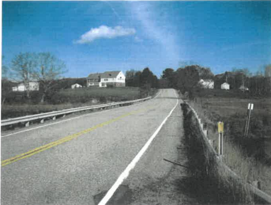
PHOTO 1 Description View of roadway facing North
