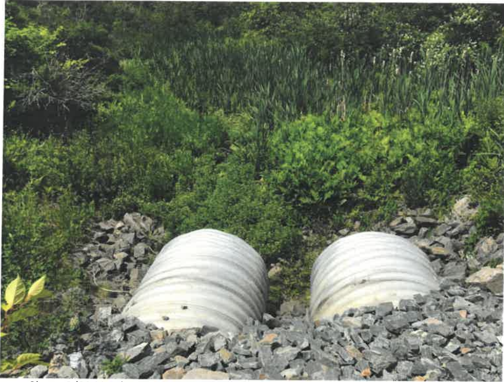
Photos 3 (06-20-18): Looking northerly from Scott Dyer Road toward the two culverts Inlets.
