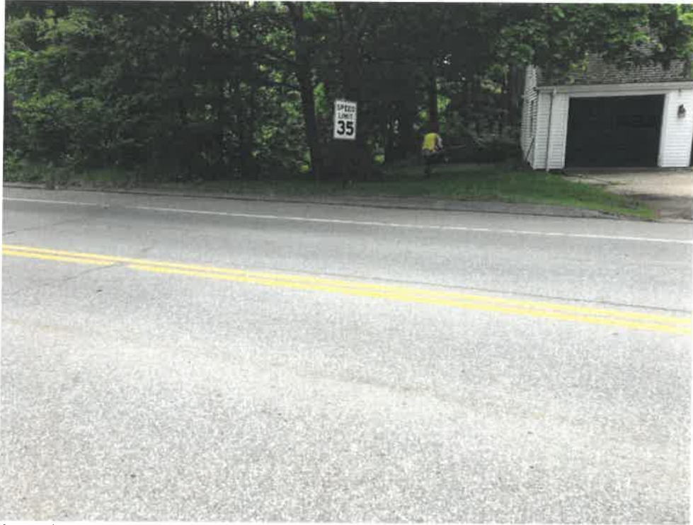
Photo 1 (06-06-18): Facing northeast at Ocean House Road (Route 77) crossing of the Trout Brook culvert.
