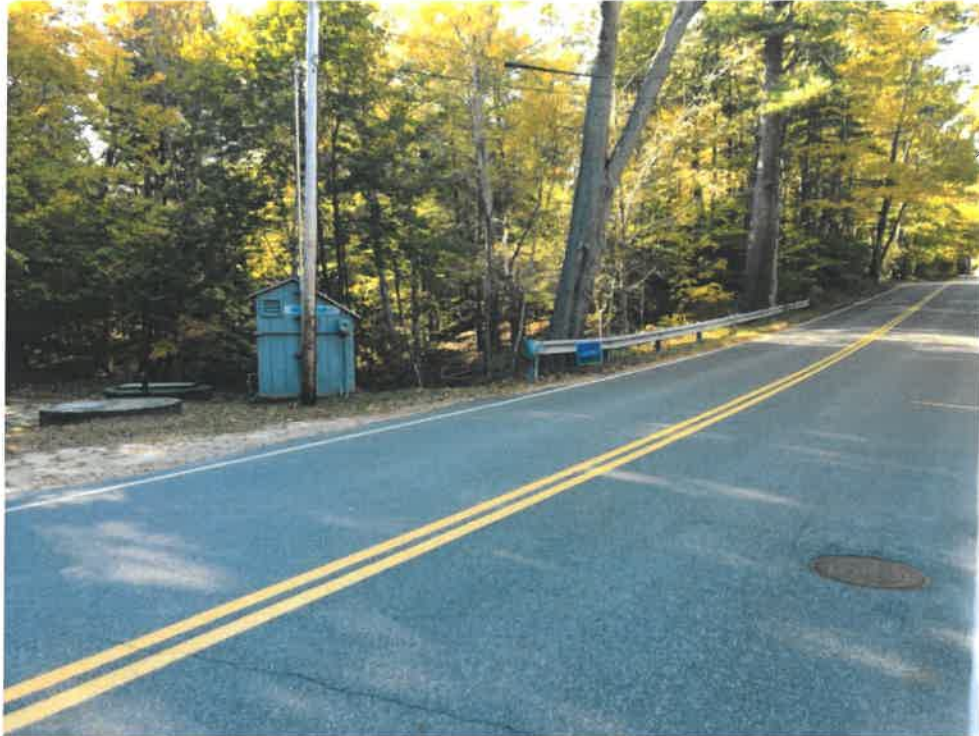
Photo 1 (10-22-18): Facing southeast at Mitchell Road crossing of Pond Cove Brook. Road is in good condition with a sanitary sewer pump station located near the brook (left hand side of photo).
