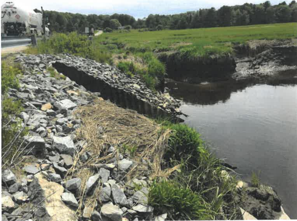
Photo 5 (06-06-18): Submerged outlet of the aluminum elliptical pipe with flared end and rip rap headwall on the west side of Sawyer Road. Quantity of rip rap appears to be sufficient on the outlet area around the culvert.
