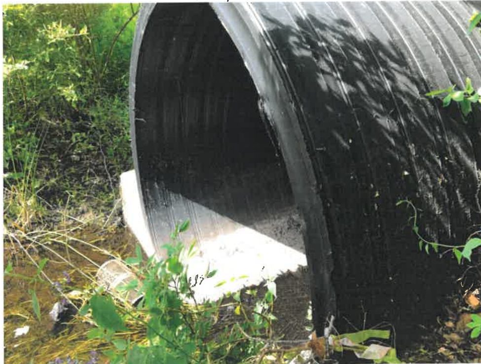
Photo 2 (06-20-18): Submerged inlet of the 70-inch high density polyethylene liner pipe within the original corrugated aluminum cross pipe. Pipe is supported on a concrete saddle.
