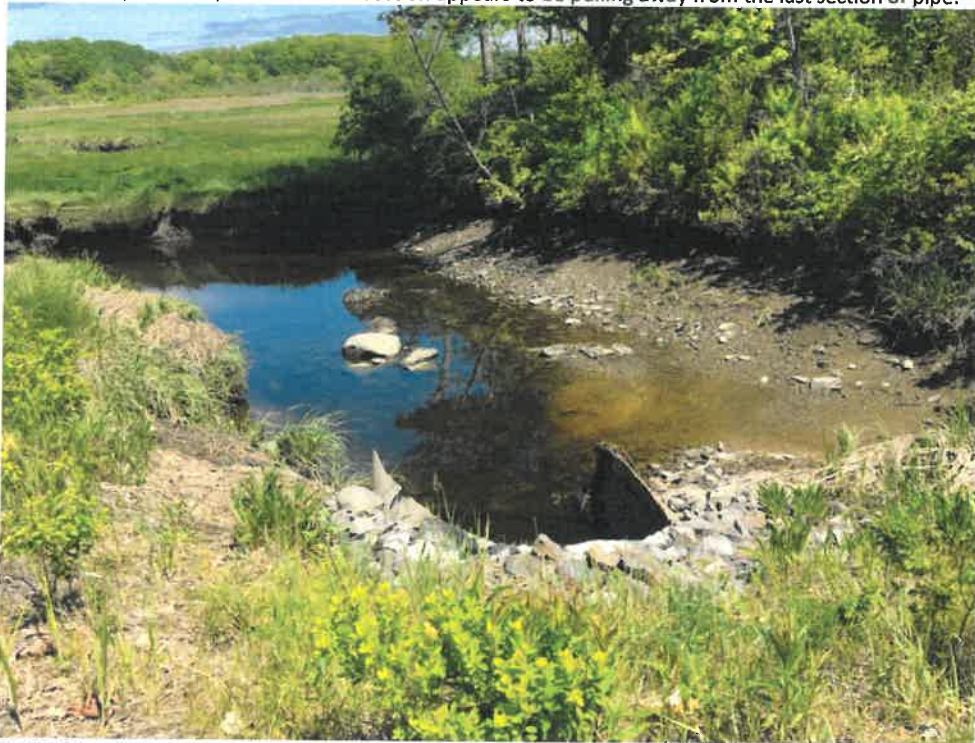
Photo 4 (06-06-18): Inlet to culvert with channel of the Spurwink River upstream of the culvert. North bank of the channel is eroded due to the sharp bend in channel just upstream of the culvert location and may need to be bolstered with rip rap armor at some point in the future.
