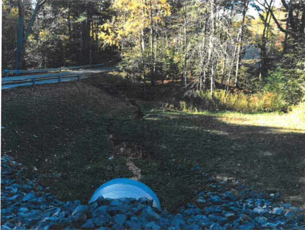
Photo 5 (10-22-18): Facing southwest at discharge flow channel of Pond Cove Brook from elliptical culvert under Hobstone Road to the Mitchell Road culvert inlet.
