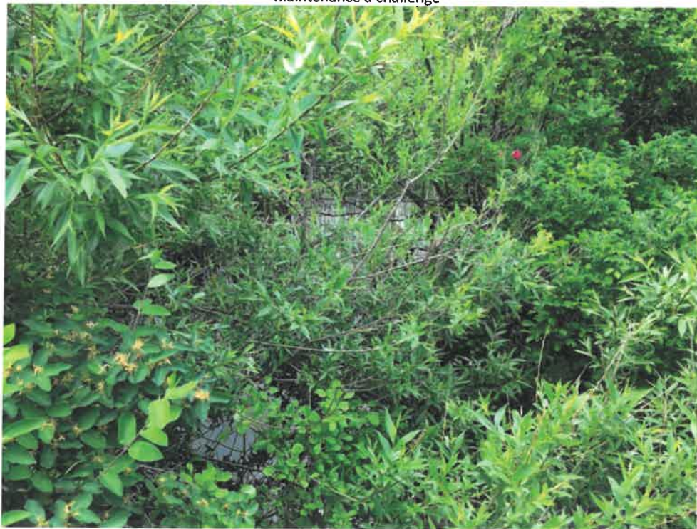
Photo 4 (06-06-18): Facing west. Thick vegetation and berm controlling ponded water up gradient of the culvert inlets.
