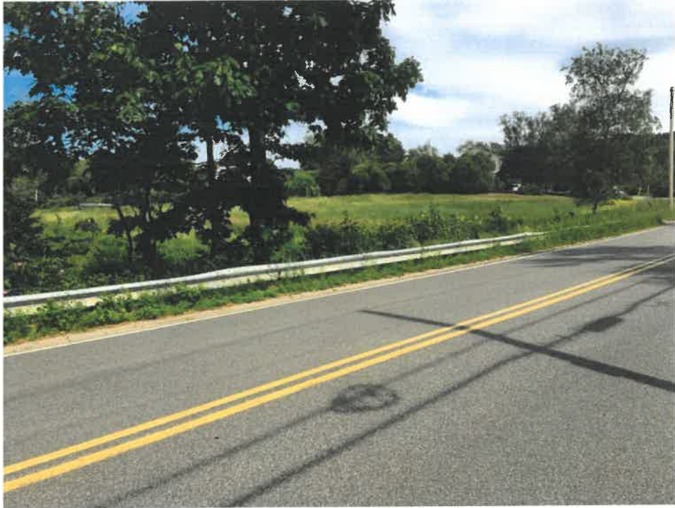
Photo 1 (06-20-18): Facing southeast at Old Ocean House Road crossing of Alewife Brook. Culvert are located relatively deep in relation to the road surface elevation with a steep roadway embankment.
