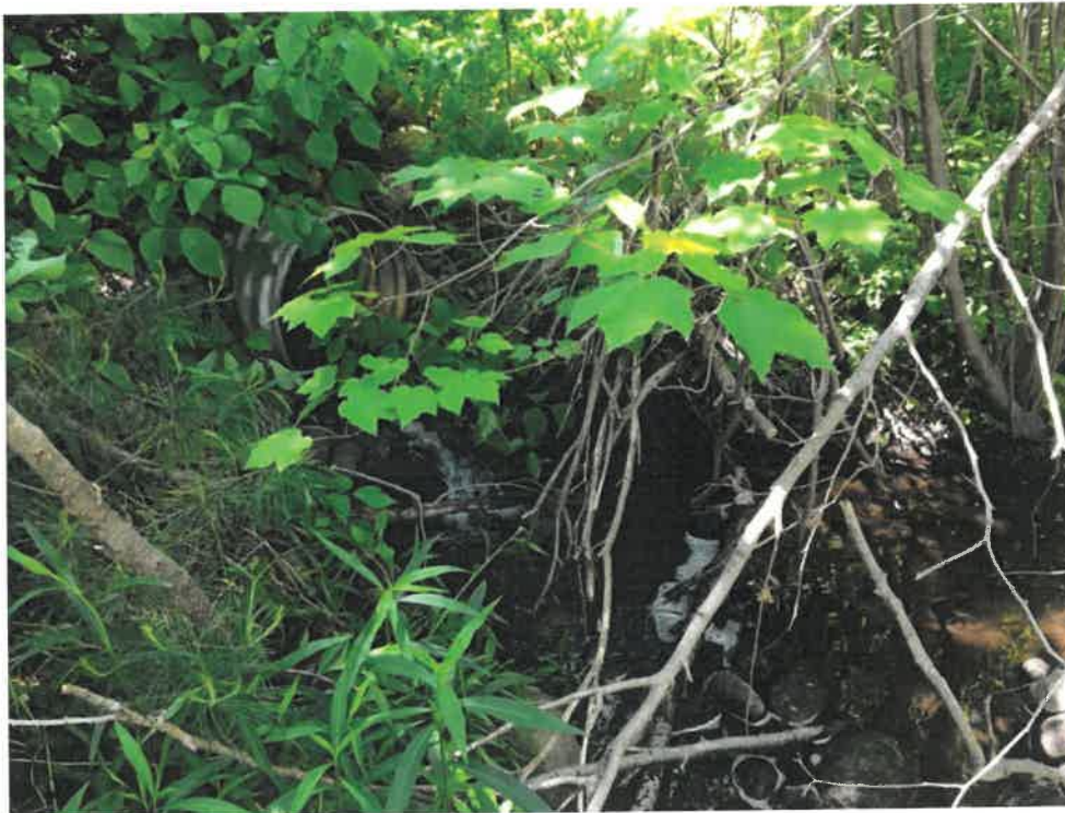
Photo 4 (06-06-18): Culvert outlet on east side of Shore Road with very thick vegetation around the culvert and in the downstream channel.
