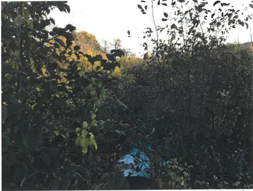
Photo 7 (06-06-18): Looking northeast at the flow from the culvert outlet on east side of Spurwink Avenue. Downstream vegetation obscured channel at the time of the photo.
