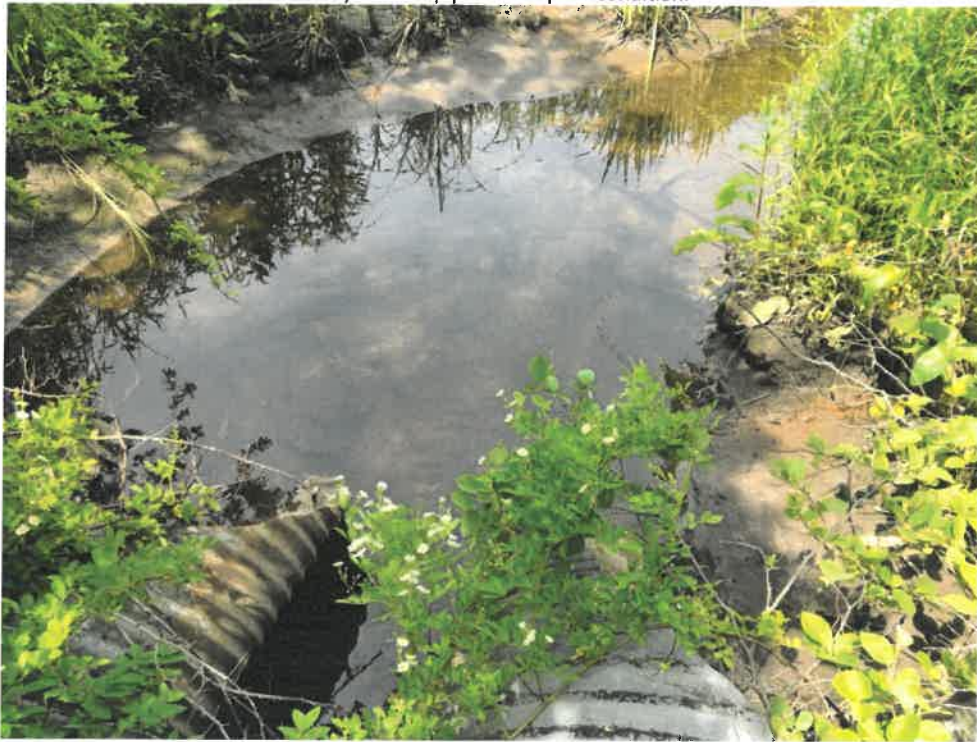
Photos 4 (06-20-18): Looking down from onto one the two culverts' inlets. Culverts' inlet area is wide just upstream from the pipes with a narrower channel further upstream flowing toward the culverts.
