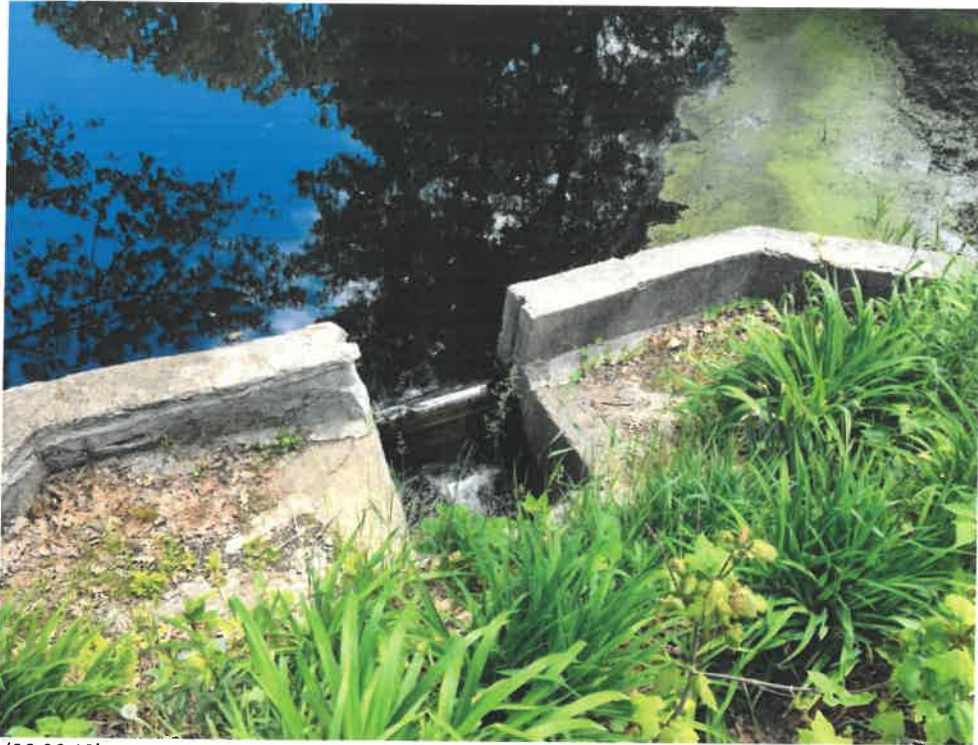
Photo 3 (06-06-18): Concrete wall with wooden board weir outlet to pond impoundment on the south side of Spurwink Avenue.
