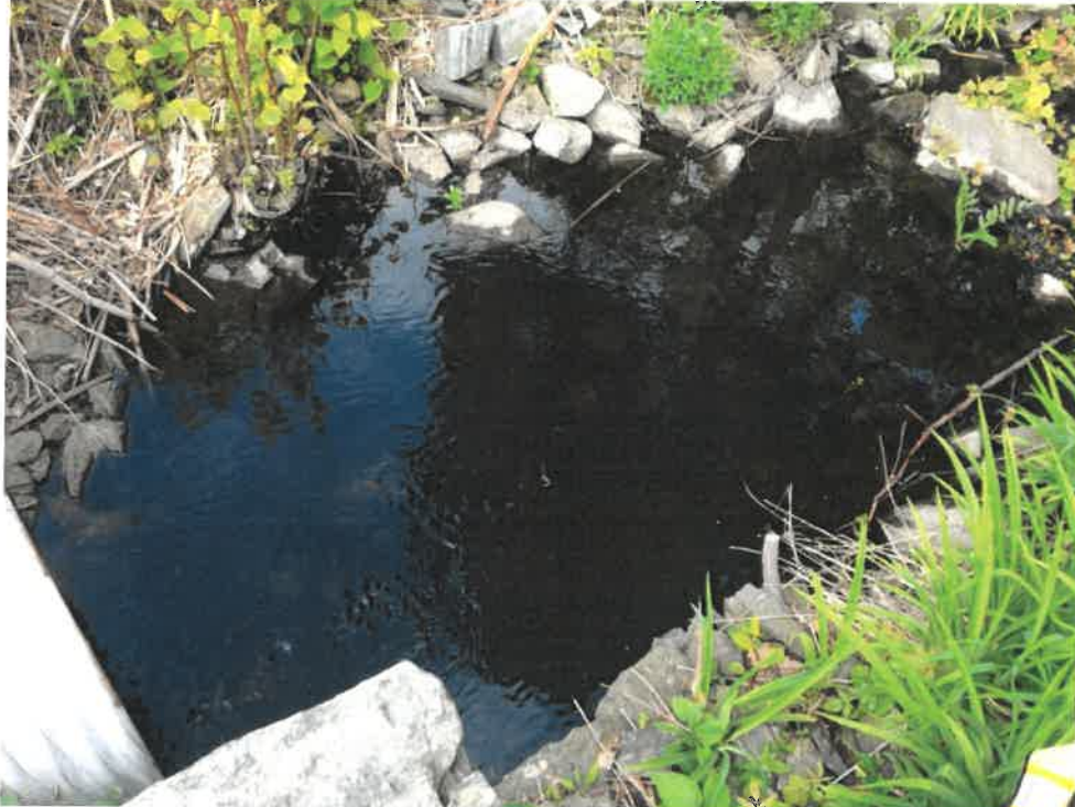
Photo 8 (06-06-18): Overhead view of culvert outlet with rip rap plunge pool apron area. Stone lined plunge pool dissipates energy of the outfall and reduces the velocity of the outflow to the receiving channel.
