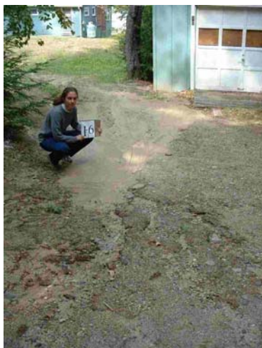
Runoff from the driveway and rooftops on this property combine to transport significant sediment into Little Sebago Lake.
