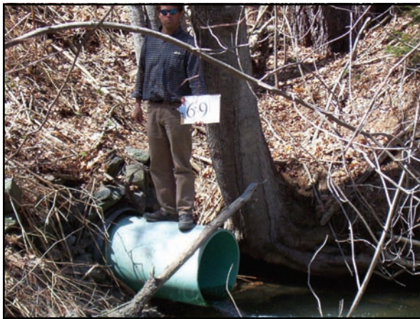
Figure 6: example of a hanging culvert.
