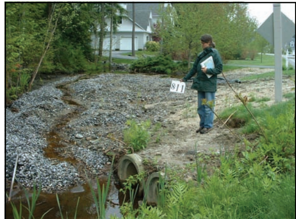
Figure 5: example of residential impact (and an inadequate vegetated buffer between pollution source and stream).
