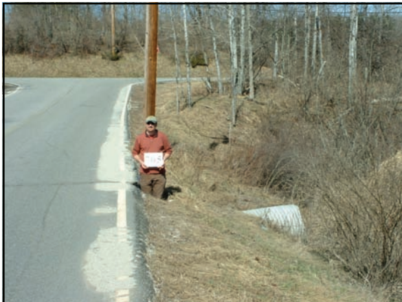
Figure 4: example of erosion on a road shoulder
