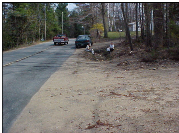
Figure 9: excess sand left on the road following a cold Maine winter.
