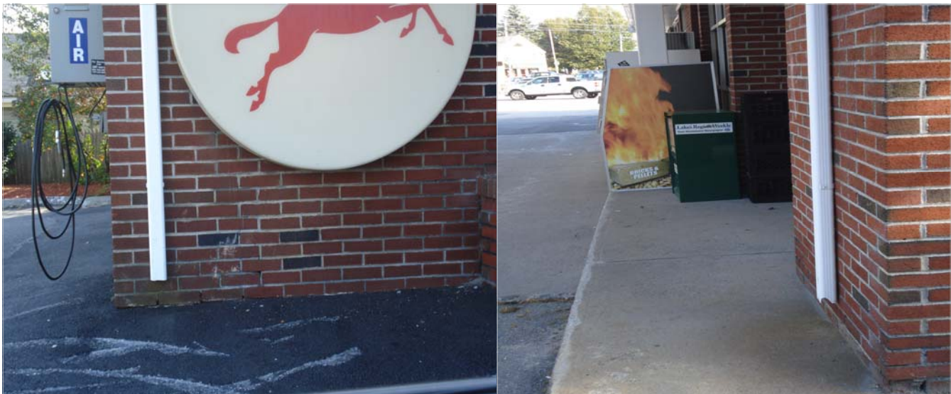
Downspouts such as these that drain to an impervious surface contributed to the designation of these properties as “potential” hotspots.
