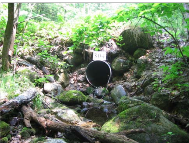
Example of a hanging culvert.
