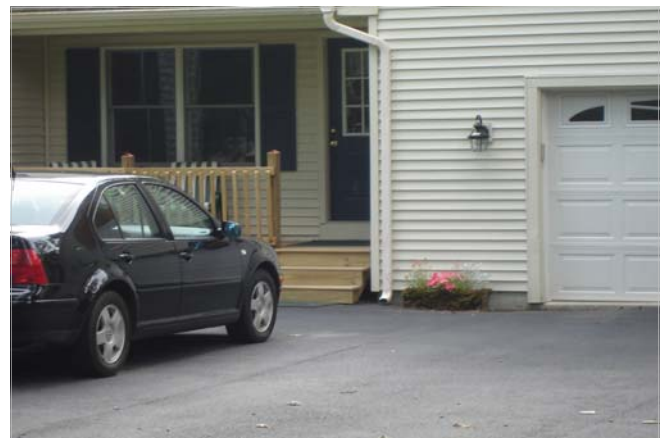
Example of downspouts leading directly to impervious surface of driveway.
