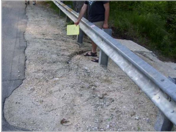
Example of erosion on a road shoulder.
