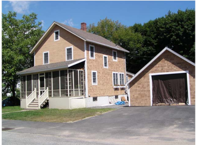
An example of a parcel with little to no landscaping and high impervious cover.
