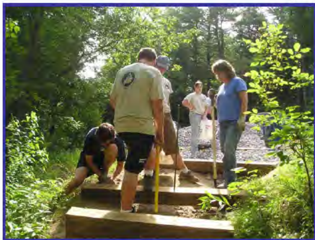
Betty Williams of the Cumberland County Soil and Water Conservation District guides the Presumpscot River Youth Conservation Corps as they install infiltration steps on an eroded trail to the Presumpscot River. Credit: Lisa Vickers, Presumpscot River Youth Conservation Corps
