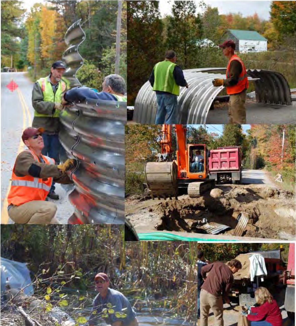
Assembly of culvert, de-watering and sand bagging and existing culvert removal.
