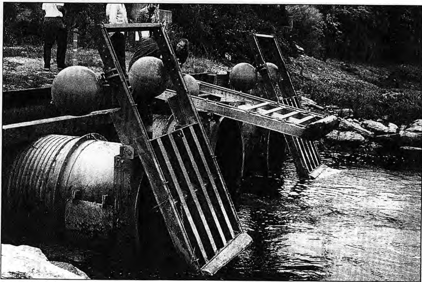
Figure 12- Self Regulating Tide Gate (after Dreyer & Niering, 1995)
