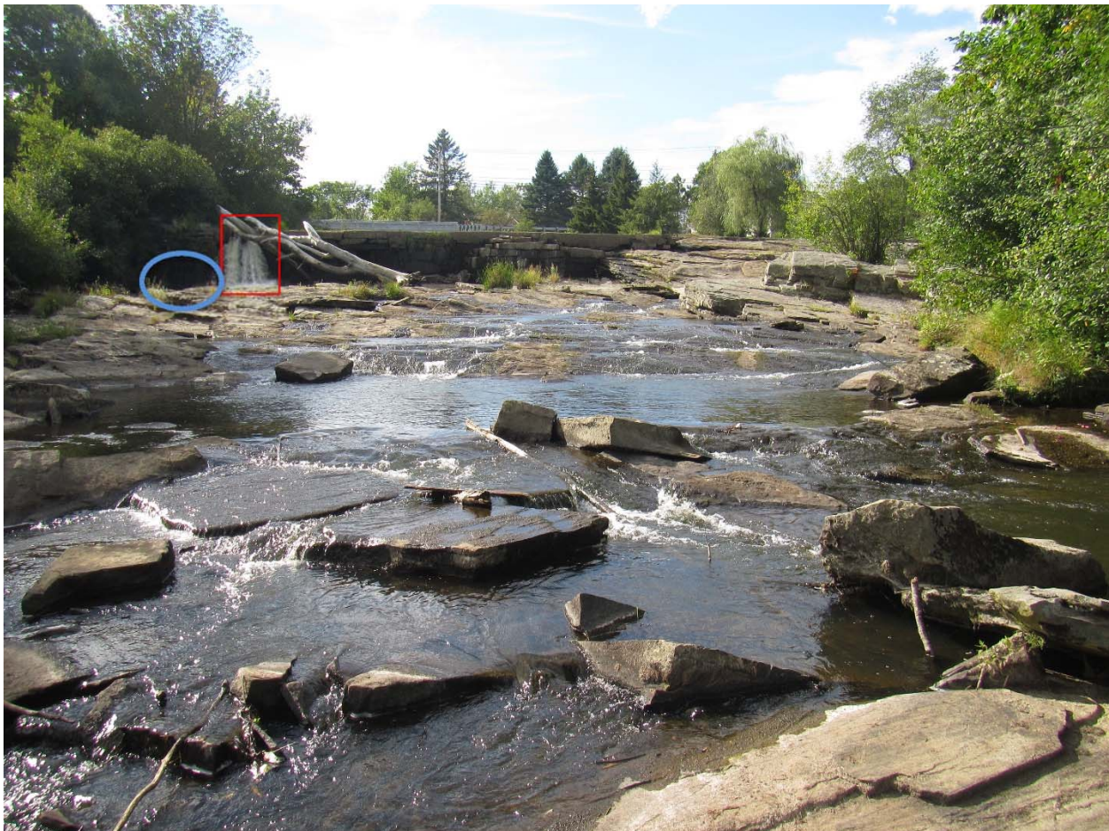
Figure 5: View looking upstream at East Elm Street Dam. Stop log weir is indicated within the red square and the fishway entrance is indicated with a blue circle. Flow direction is towards viewer.
