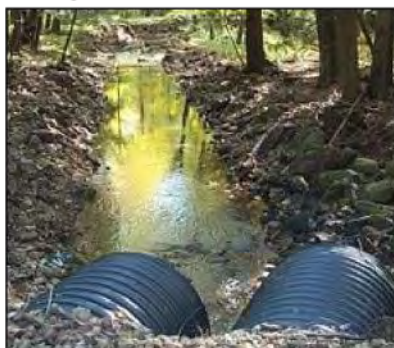
Misaligned Culvert
