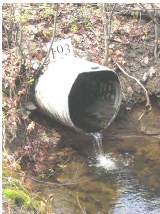
Hanging culvert flowing to Stroudwater River
