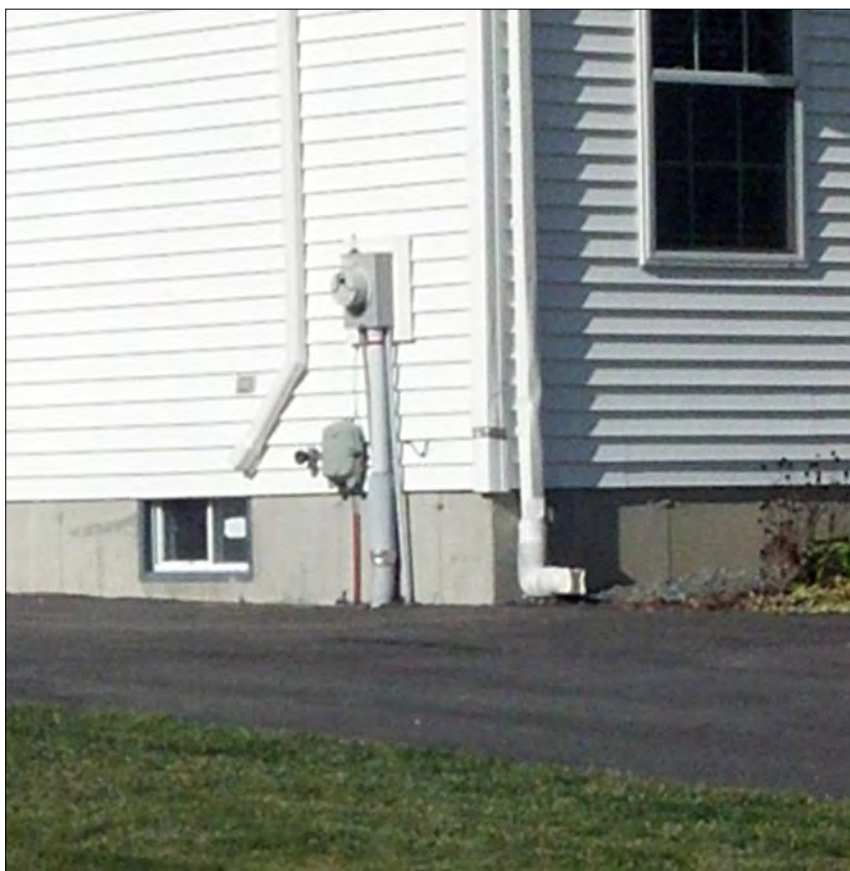
A gutter downspout empties onto a paved driveway. Downspouts should be directed to vegetated areas so the water can soak into the ground.
