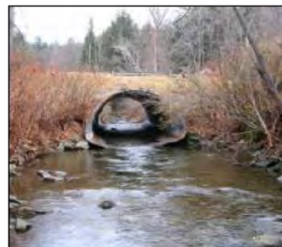
Undersized Culvert
