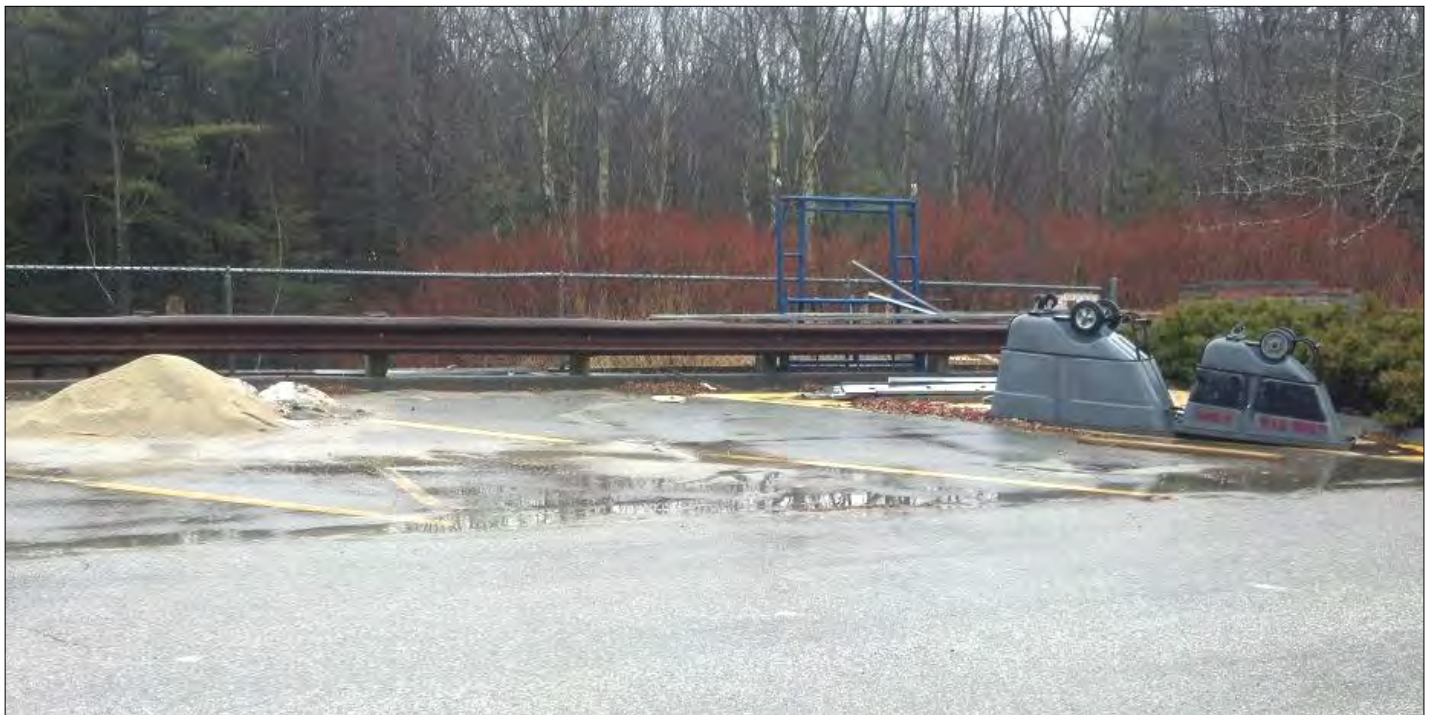
A sand pile washing into a catch basin in the Stroudwater River watershed may contribute pollutants to the River.
