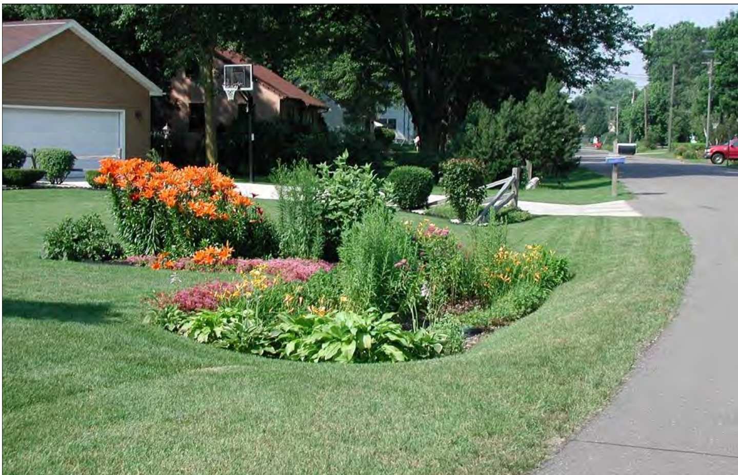
Rain garden installed at residential property in Minnesota. (Source: www.apwa.net )
