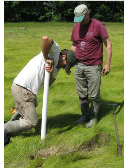
Photo 3. Installing a deep water monitoring well.
