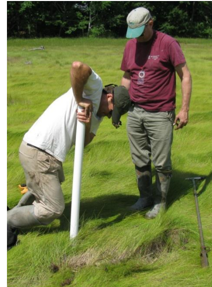
Photo 2. Installing a deep water monitoring well.
