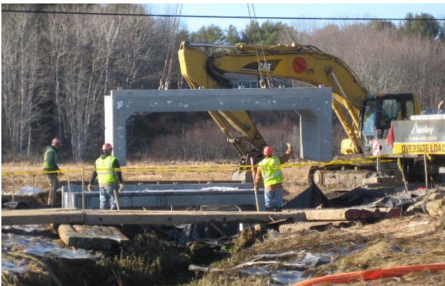
Figure 1. Installation of open bottom concrete box culvert at the lower site (9079, left) and embedded concrete round pipe at the upper site (9078, right).
