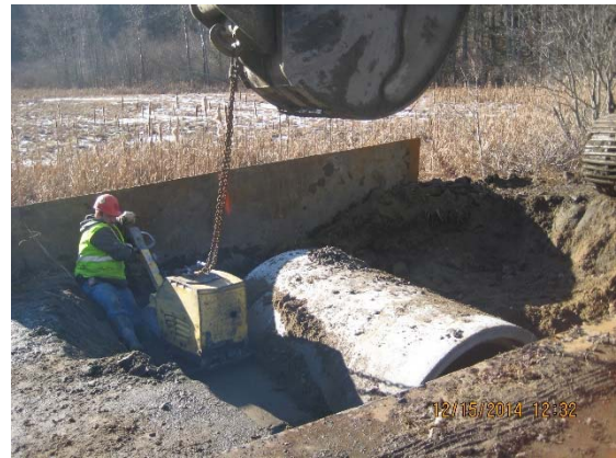
Figure 1. Installation of open bottom concrete box culvert at the lower site (9079, left) and embedded concrete round pipe at the upper site (9078, right).
