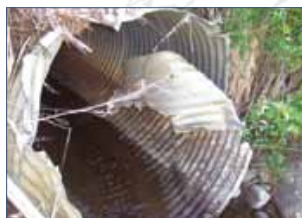
damaged culvert
