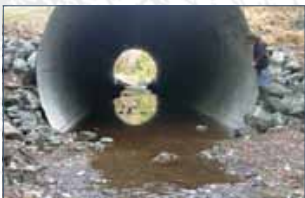
culvert properly embedded into streambed
