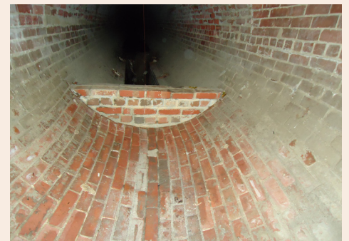
Weir inside a large Portland CSO. Weirs prevent CSO discharges under low-flow conditions. (Photo: PWD)
