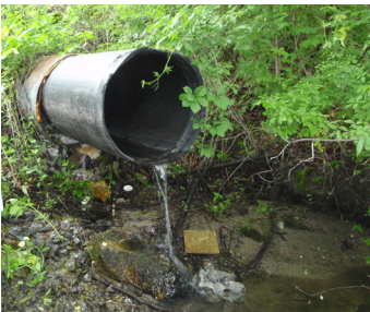
This perched, slip-lined round culvert obstructs movement of fish and other aquatic organisms. (Photo: Maine Stream Habitat Viewer)
