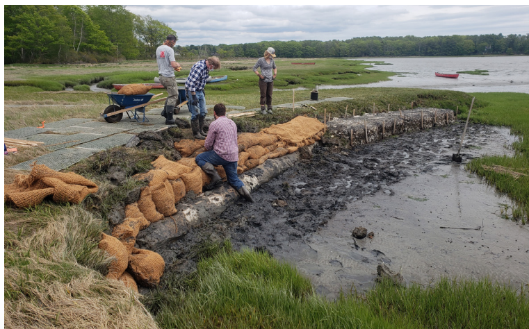
In a pilot project to test the use of natural elements to protect against shoreline erosion, a team led by Maine Geological Survey installed "living shorelines" at three sites around Casco Bay. (Photo: Maine Geological Survey)
