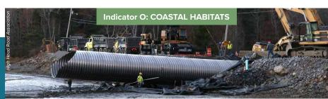
Many tidal marshes have been degraded or converted to freshwater wetlands by roads, railways, dams, and dikes. Replacement of undersized culverts in Brunswick and Harpswell has restored tidal flow to 115 acres of marsh. See map below.
